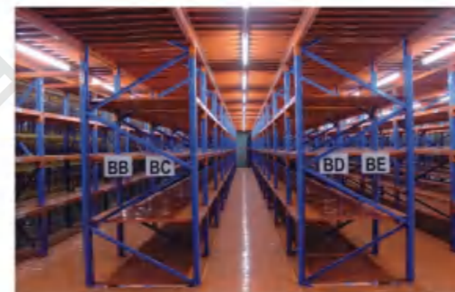
二層擱樓式貨架案例 Case of 2 layers mezzanine racking
